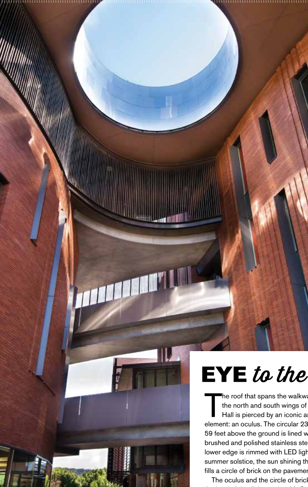
The architects of McCord Hall used the oculus to produce a circle of light on the patio during the summer solstice.
